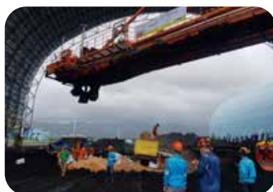
Uji Cofiring Biomassa Biomass Co-firing Test
